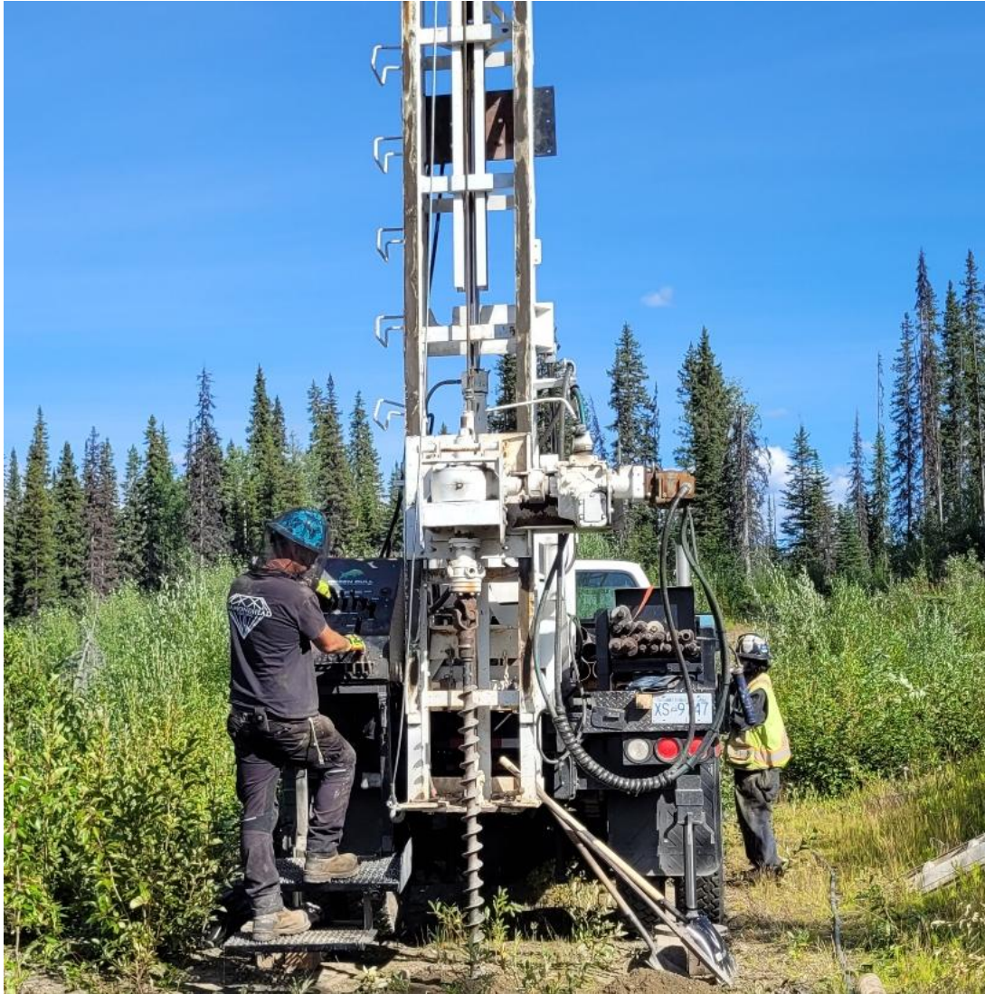
Figure 3: Photo Auger drilling at Camp north area
